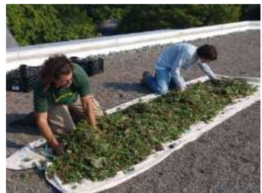
Planting a green roof at Swarthmore College, a PERC member school.
